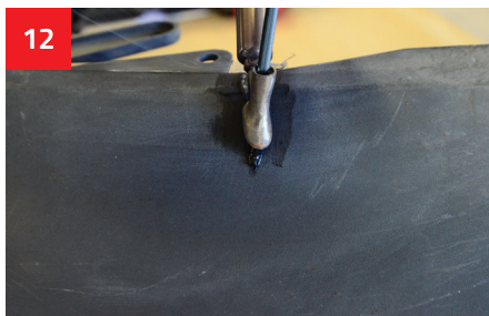
Set the binding material in the damaged area and even up the surface.
