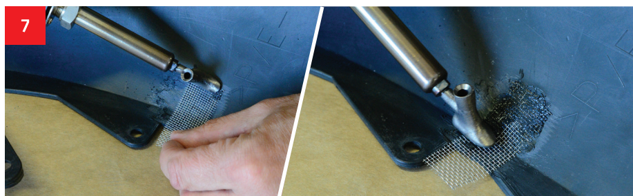
7 Embed the aluminum mesh in the damaged element on the inner side of the damage with the welding tool.
